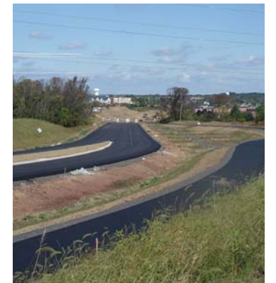
The Parkway and Shared Use Path in Section 701 are virtually finished.
