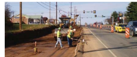
Construction continues on the widening of Horsham Road.
