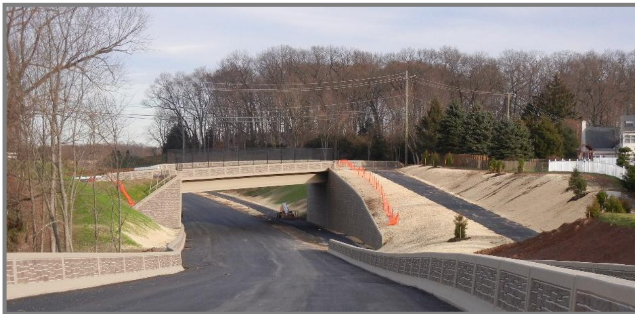
Photo 5: The Wells Road Overpass
