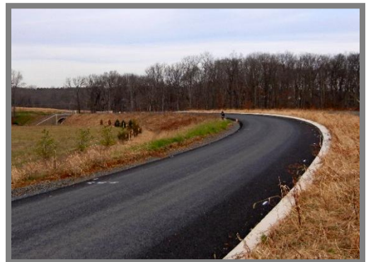
Photo 2: A paved section of Parkway north of Horsham Road
