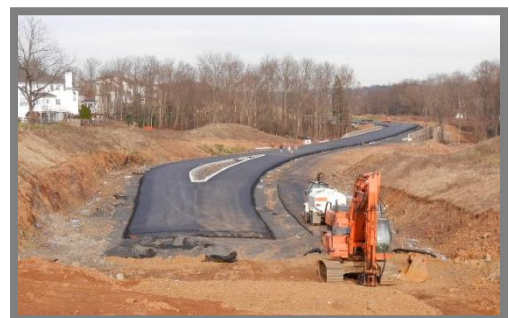
Photo 3: Paving in place just north of Pickertown Road
