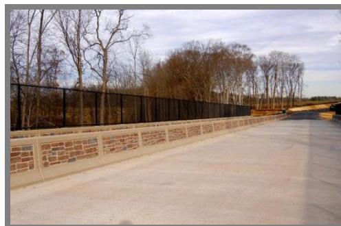
Photo 4: The Parkway bridge over Neshaminy Creek
