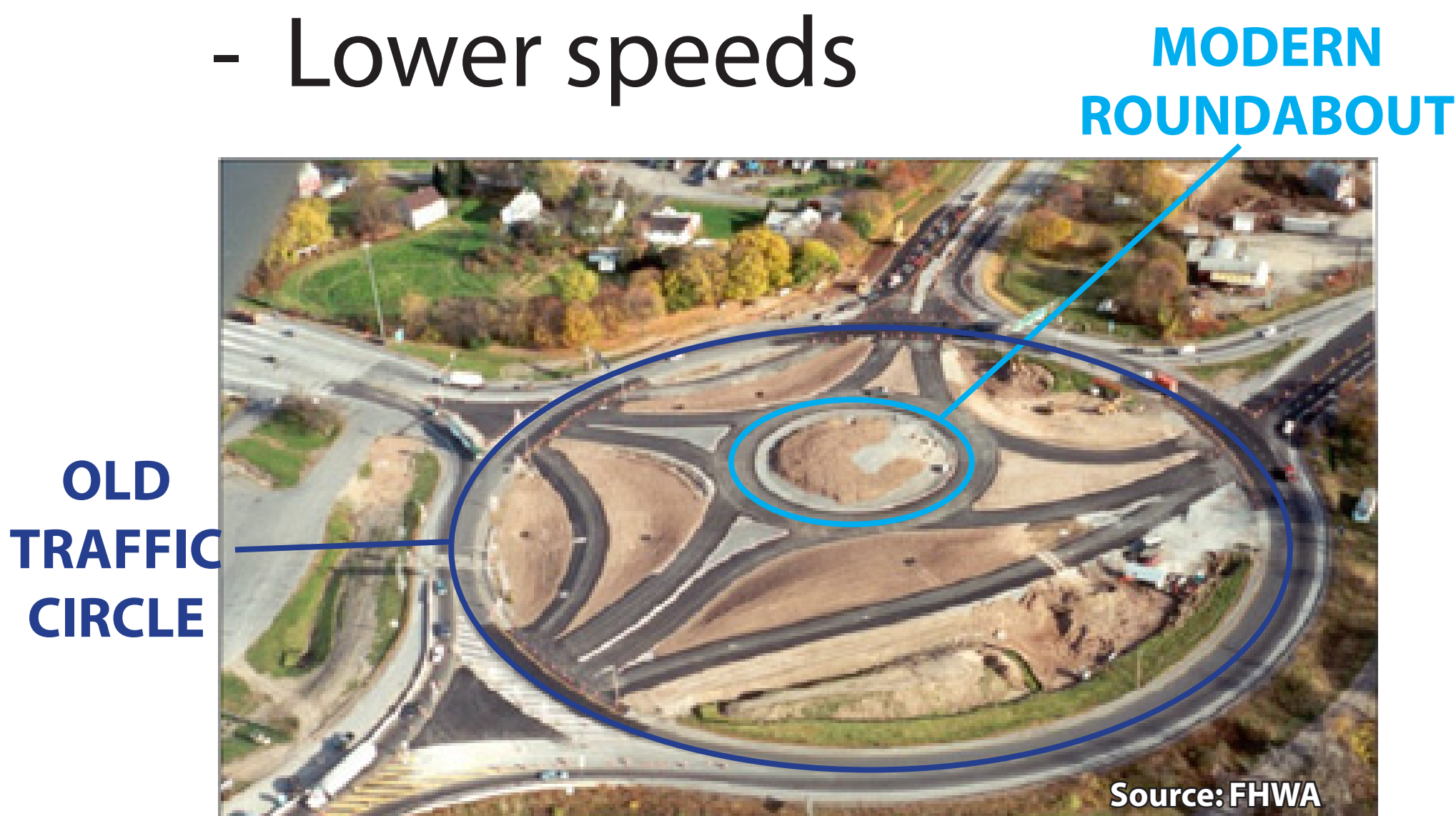
A modern roundabout was constructed in Kingston, NY to take the place of an existing traffic circle.
